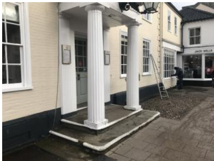
Main Entrance Steps
