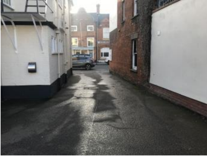
Entrance To Car Park From Road 1
