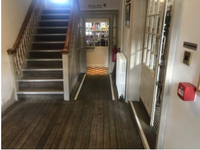
Stairs To First Floor 1
