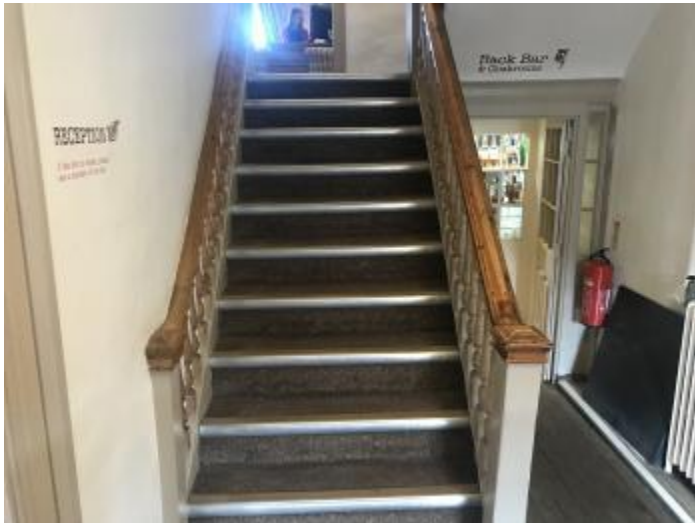
Stairs To First Floor 2
